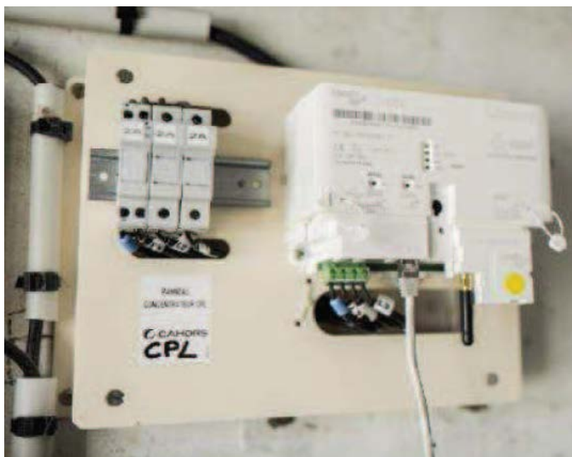
Figure 32: Installed Concentrator
