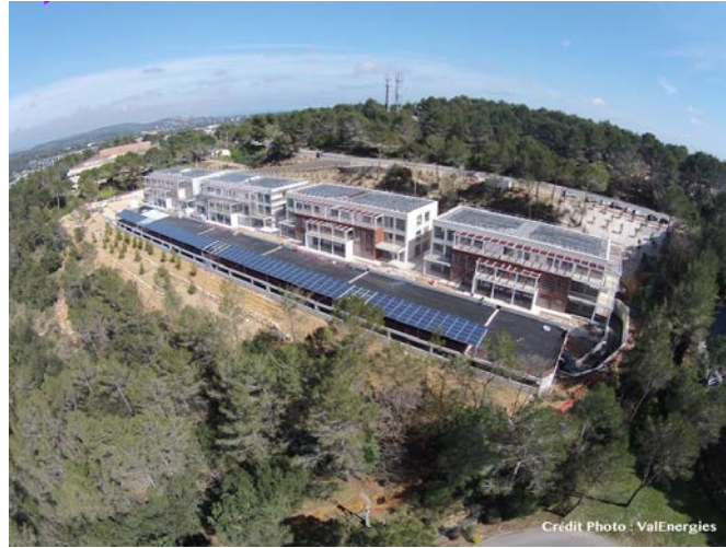
Figure 6 – Collective self-consumption of PV in ValSophia, a group of 4 office buildings equipped with PV systems (238 kWp)
