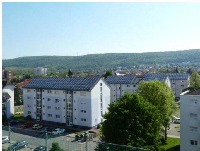
Figure 4 - Collective self-consumption in the “Neue Heimat” Cooperative Family Home equipped with 7 PV systems (445 kWp)
