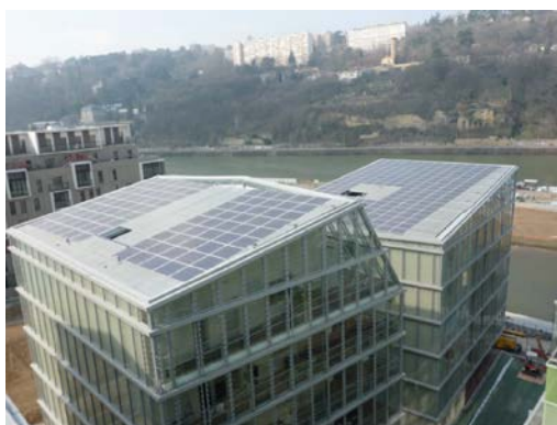
Figure 9 - Architecturally integrated PV systems of A block (79 kWp)
